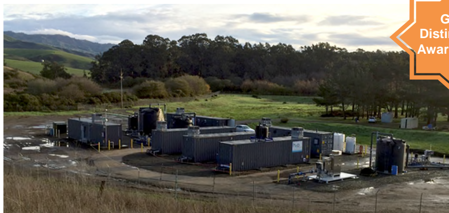
Cambria, California – UF/RO 587 gpm
