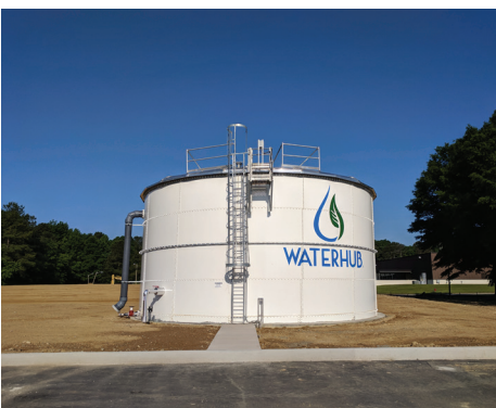
Universal platform for support and interchanging membrane modules at Virginia WaterHub™
