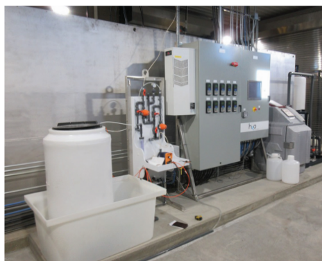
Figure 2: Packaged Plant MBR System at Craig WWTP
