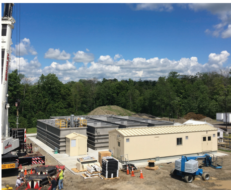
Diesel Engine Manufacturer's site under construction
