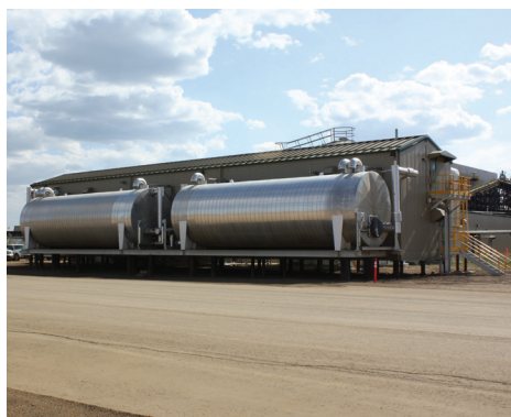
Construction of the building for Oil & Gas Client
