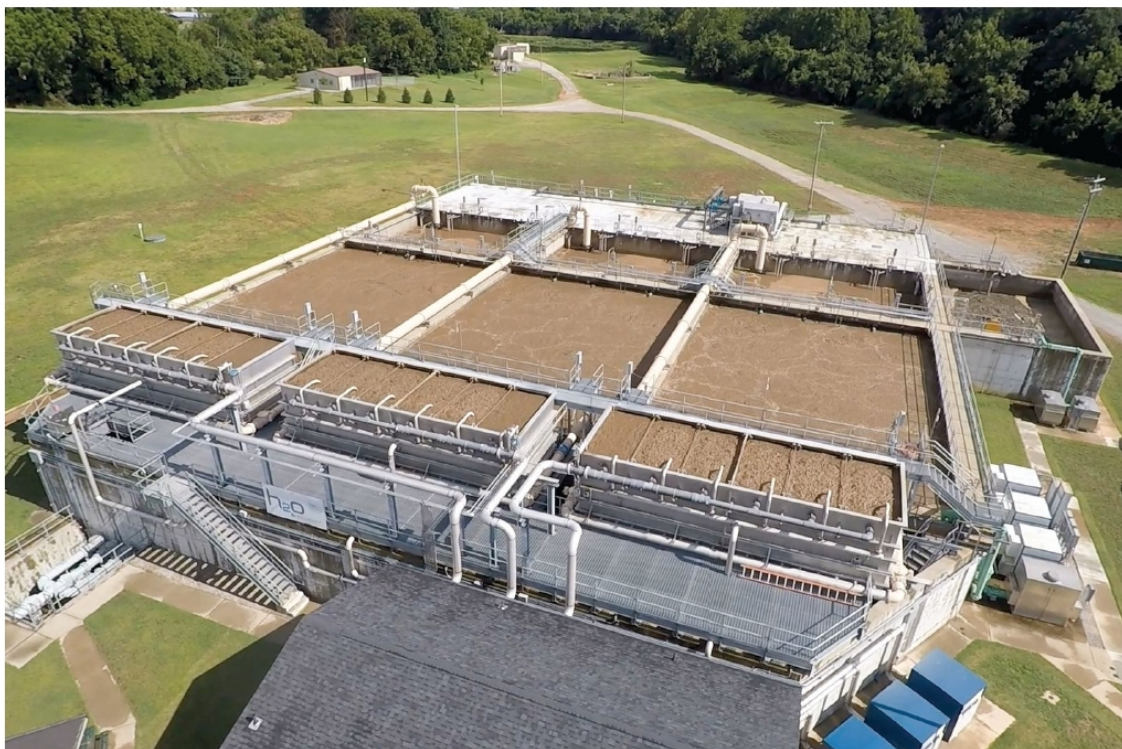
The Decatur, Arkansas, Wastewater Treatment Plant became the first membrane bioreactor (MBR) plant in the state. The MBR design chosen is open-source and modular, which allowed the city to source membranes for the reactor from multiple manufacturers and keep options open for future upgrades.
