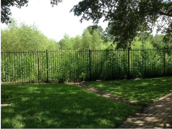
Old picture taken above spillway drain into Barker Reservoir
