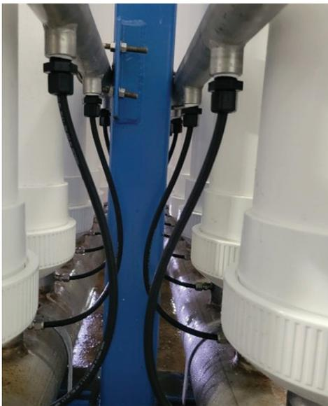
Installation of the UF membrane modules
