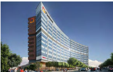
Piedmont Hospital, Atlanta, GA, USA.
