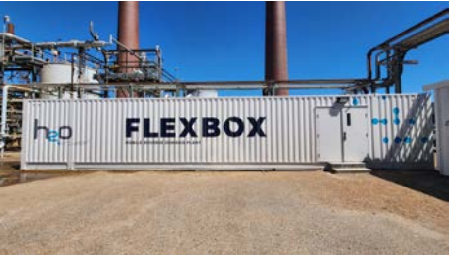
Flexbox RO on Oil & Gas extraction site
